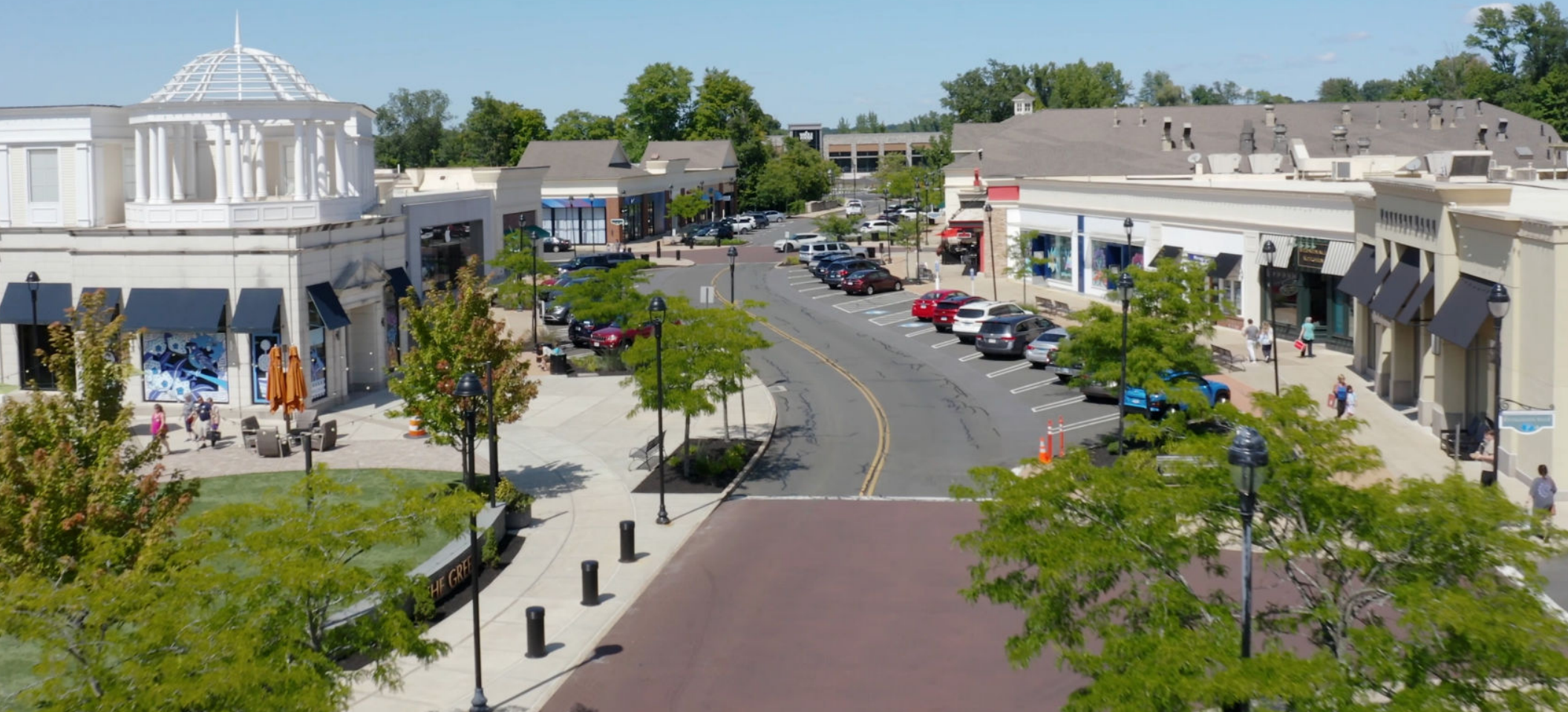
The Shops at Evergreen Walk is located along the Buckland Road, just off the interchange between I-84 and I-291. A prominent mixed-use lifestyle project, Evergreen Walk provides the only walkable “downtown” streetscape in the market.
